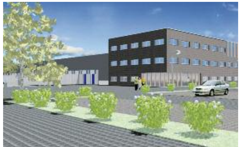
Wincanton operates from four sites in the Netherlands, including its new 7,500 m 2 building in 's-Heerenberg
